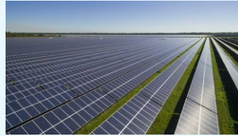
Solar Panel Fields
