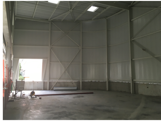
(b) ENAC flight hall under construction, to be finished by November 2017.
